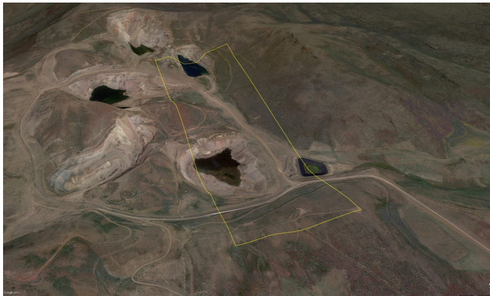
Fig 3. Current view (2015) of the Mule Canyon Mine, showing the pre-mining biogeochemical survey area (1986).
