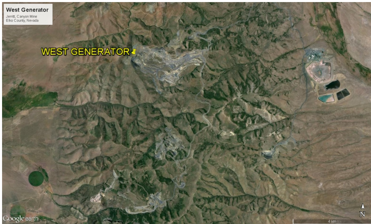
Fig 2. Location map of West Generator in the Jerritt Canyon Mine complex, Elko County, Nevada.
